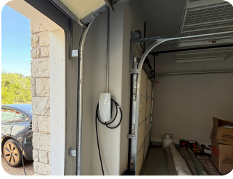
Up and over. Conduit run above the garage door to reach the far wall.
